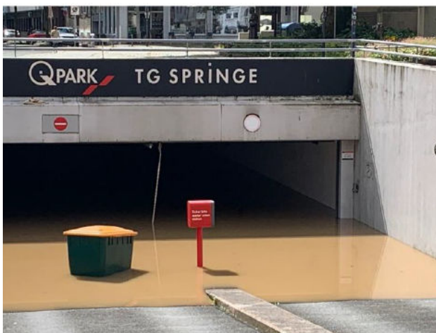
Figure 12: Flooded car park in Hagen, Germany
